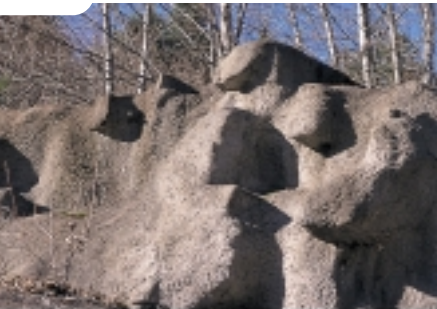
BELOW : Slope stabilization
